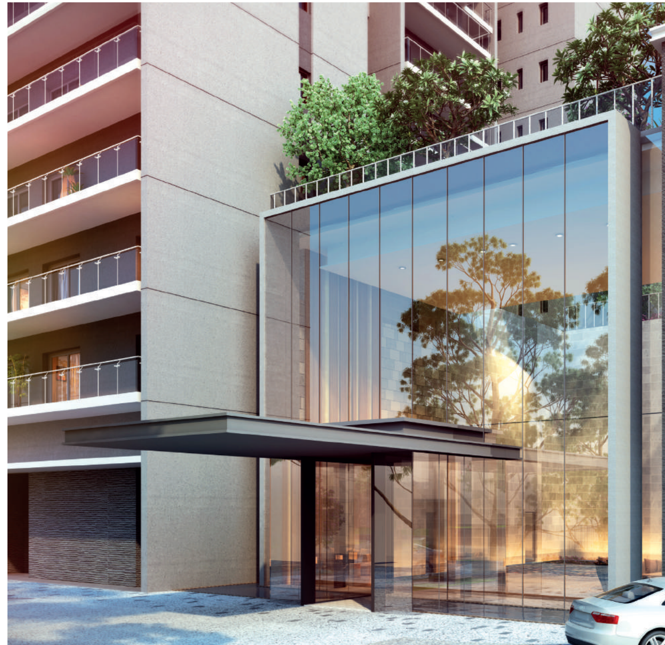
Tower C Drop-Off •
